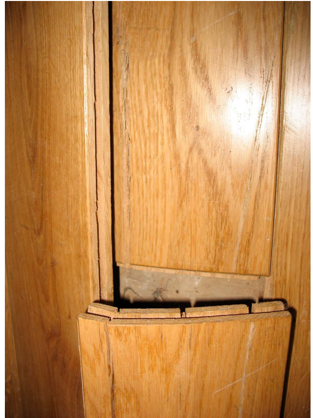
Floorboards that have been tightly re-fixed without sufficient drying have bowed.
