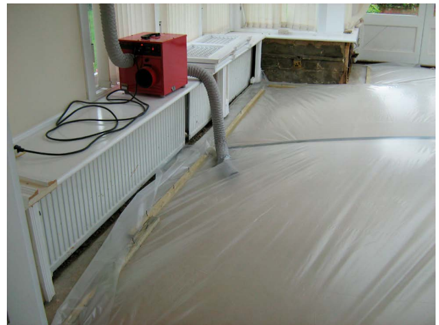
A desiccant dehumidifier being used with polythene sheeting to isolate a particular area.
